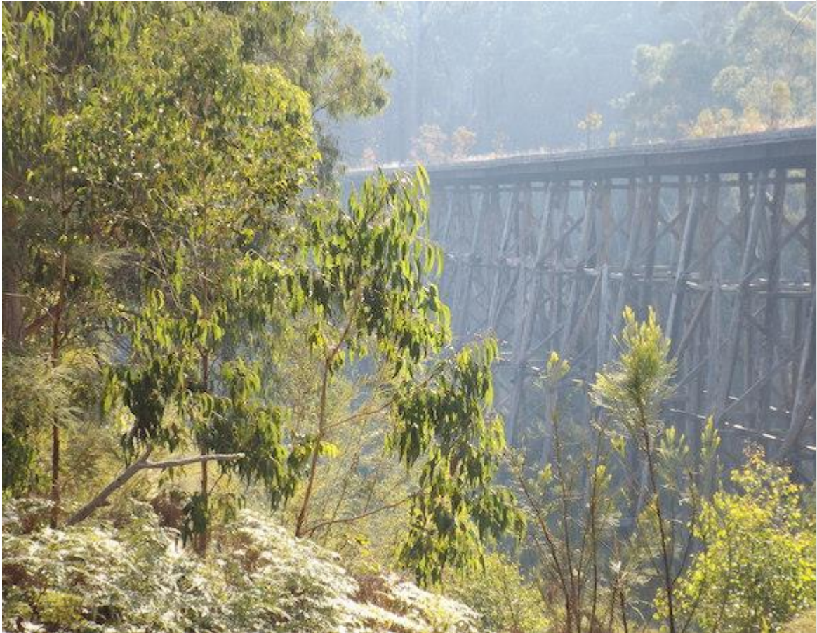
Stony Creek Trestle Bridge. Photo Ross
