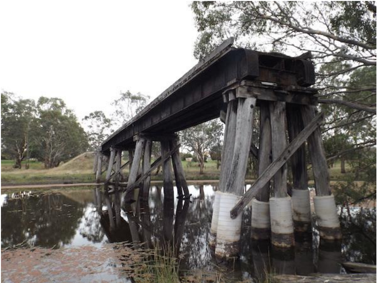
Disused railway bridge, Cavendish. Photo Ross Byrne
